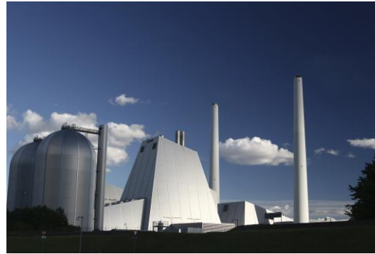
Power Gen.: lube and off-line filtration for engines, lube and cooling for turbo machinery, oil jacking.
